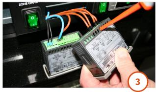
Removing the cables one by one, rewire into the new Dixell controller terminals respectively, ensuring a secure connection.
